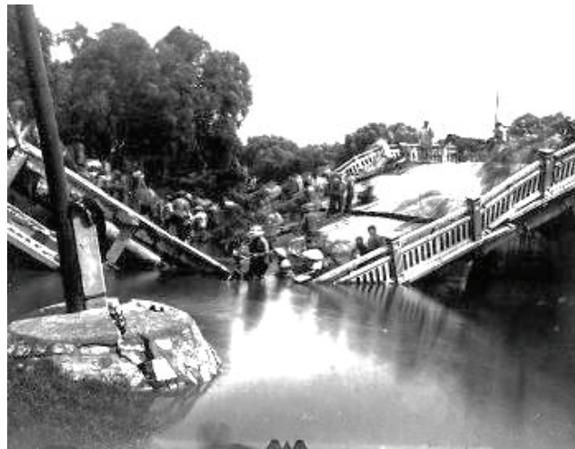
Figura I 13-2: Sismo de Tangshan: El colapso del Chengli Bridge. (Fuente: Wang Fang, State Seismological Bureau of China en http://earthquake.usgs.gov/earthquakes/world/events/1976_07_27_eib.php )
