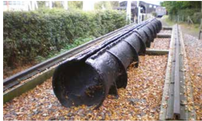
Figure 1 - The track with atmospheric propulsion in the center, South Devon railway corridor 6
