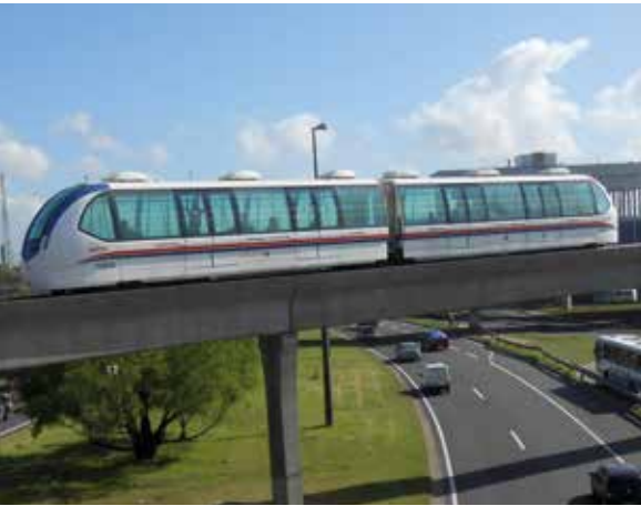
Figure 5 - Aeromovel technology operating in Porto Alegre, Brazil 14
