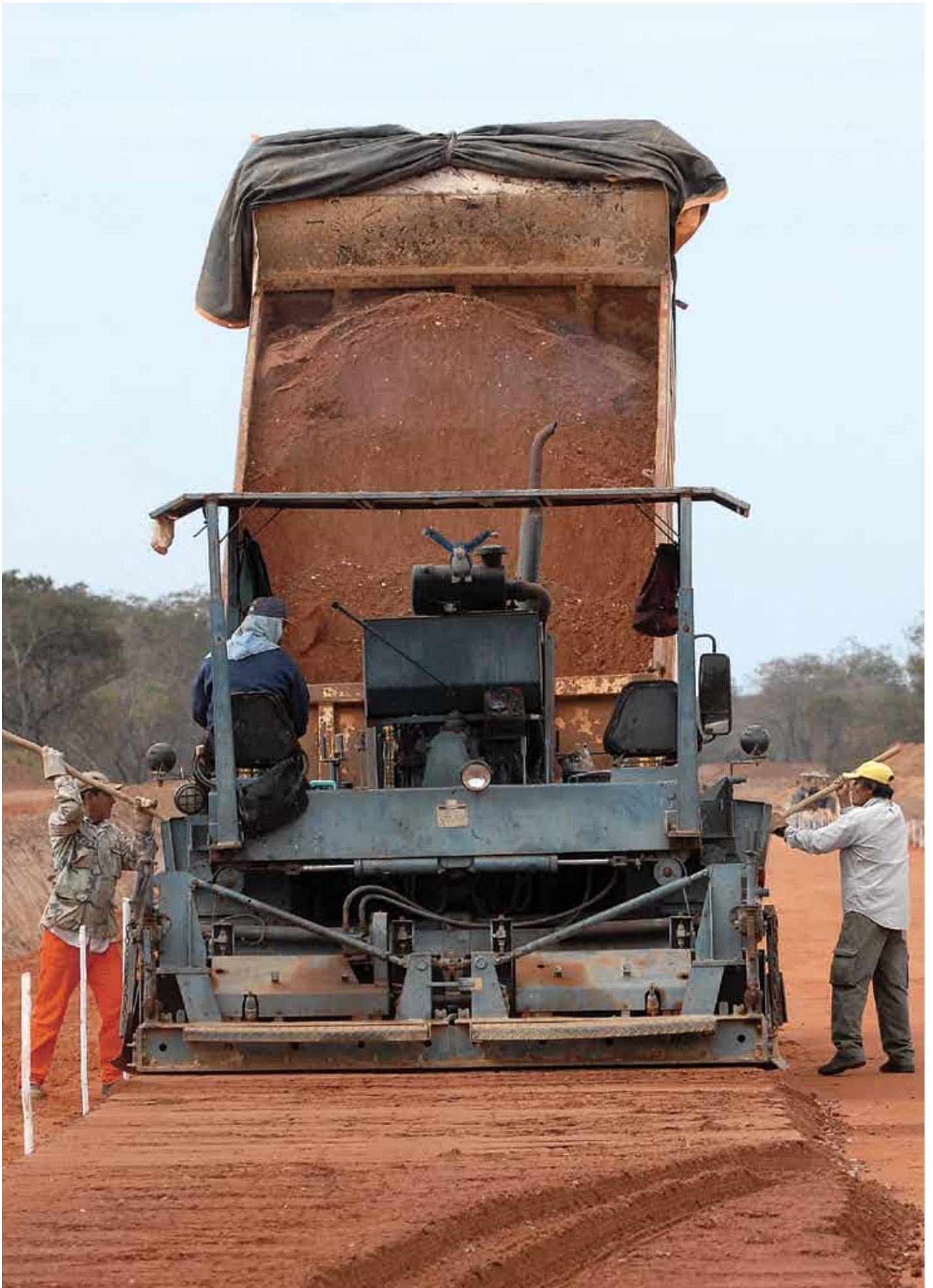
Construction in the Santa Cruz-Puerto Suarez Road Corridor. Bolivia.
