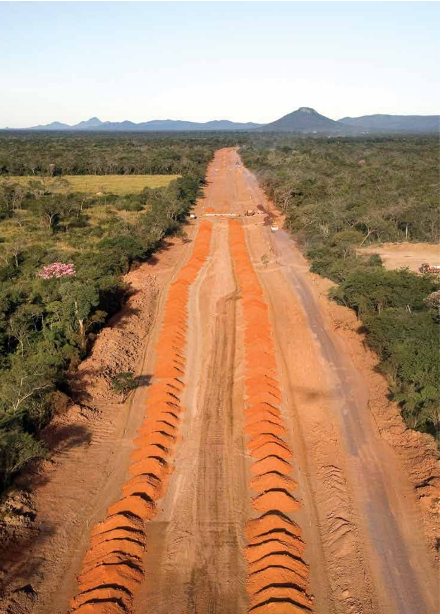
Works East of San Jose. Santa Cruz-Puerto Suarez Road Corridor. Bolivia.
